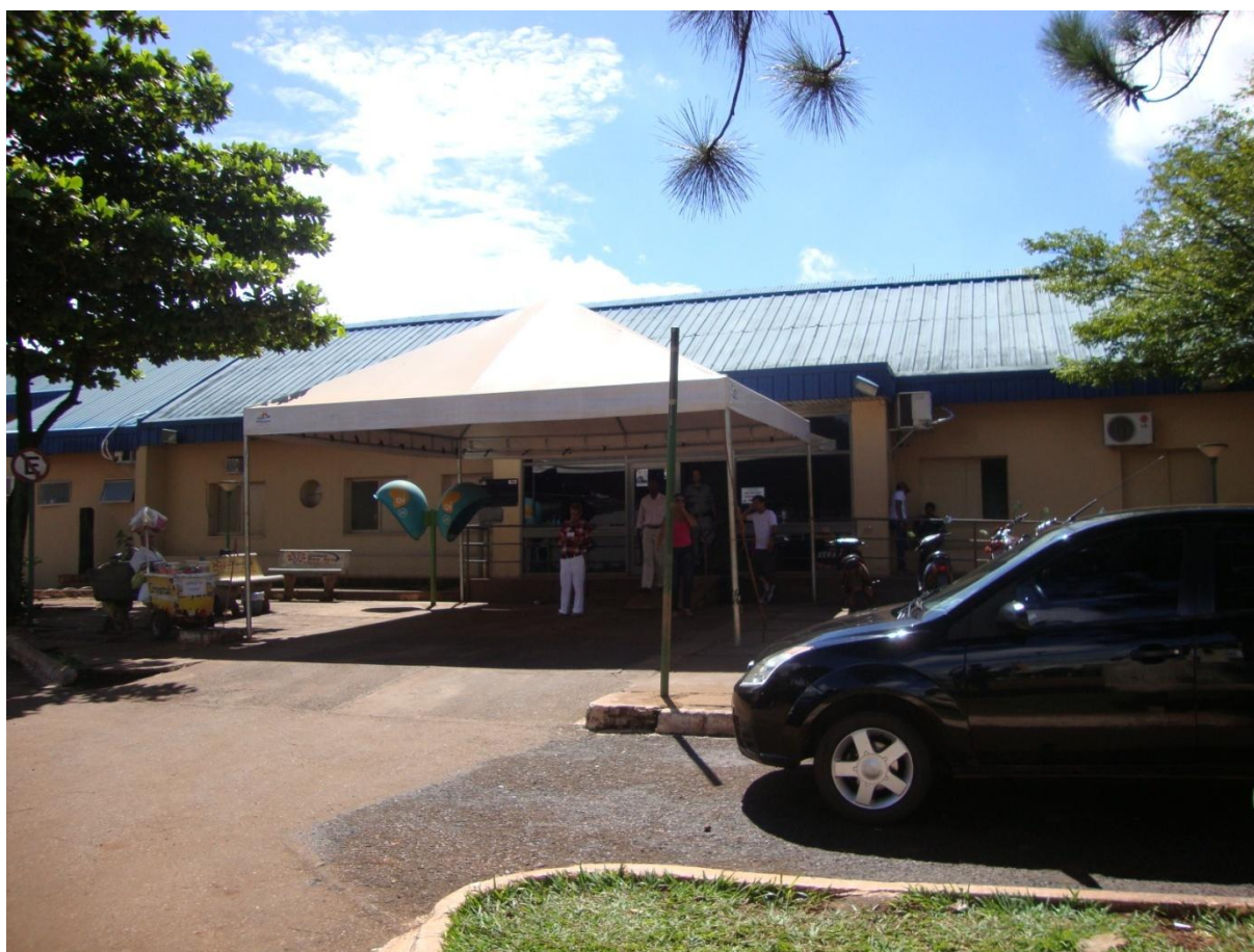
Figura 37: Hospital Municipal de Rio Verde – GO
